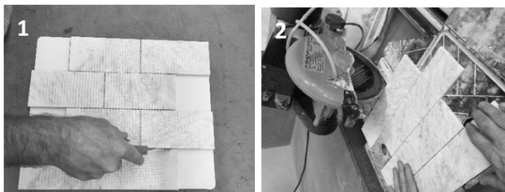
2. **Images 1-2.** If you need to cut a mosaic sheet, cut from the mesh from the back with a utility knife. As much as possible, make sure the mosaic tile sheets are cut between tiles. It is difficult to cut individual tiles. Use a wet saw with a diamond blade to cut through the tiles.
