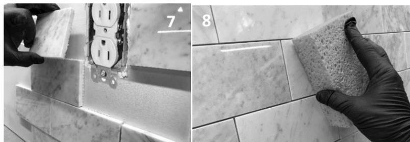
6. Once the mosaic tile installation is completed, it may be necessary to install an electrical box extender (found at your local hardware store) around electrical sockets or switches to allow the electrical plate to sit flush against the tile. **Ensure that the power supply to the outlet is turned off** when installing an electrical box extender, and follow the manufacturer's installation instructions or consult your local electrician.
