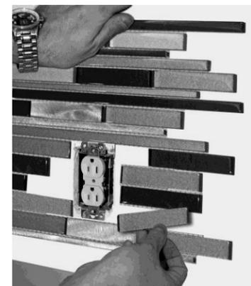
6. Once the mosaic tile installation is completed, it may be necessary to install an electrical box extender (found at your local hardware store) around electrical sockets or switches to allow the electrical plate to sit flush against the tile. Ensure that the power supply to the outlet is turned off when installing an electrical box extender, and follow the manufacturer’s installation instructions or consult your local electrician.
