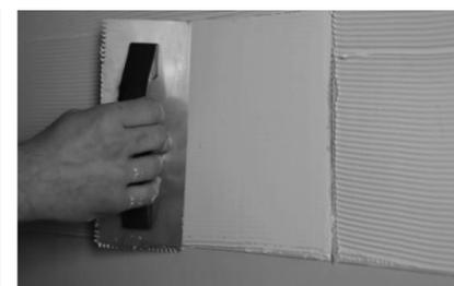
3. Apply setting materials to the substrate using the notched side of a V-notched trowel. Using the flat side of the trowel, smooth out all ridges to achieve a consistent, even 3 mm (1/8 in) coverage.
