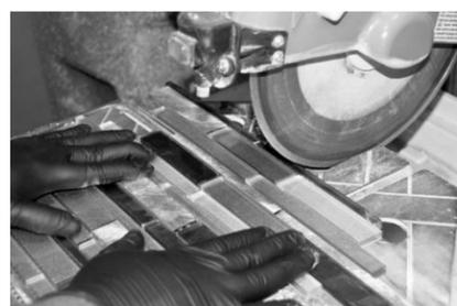
2. If you need to cut a mosaic sheet, cut from the back with a utility knife. As much as possible, make sure the mosaic tile sheets are cut between tiles. It is difficult to cut individual tiles. Use a wet saw with a diamond blade to cut through the tiles.
