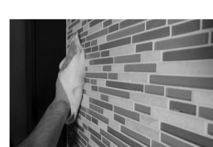
8. Natural stone should be sealed prior to grouting. A premium penetrating sealer is recommended for a natural look. Please refer to Sealer Manufacturer’s recommendations for application instructions. Ensure that you only apply the sealer onto the stone.
