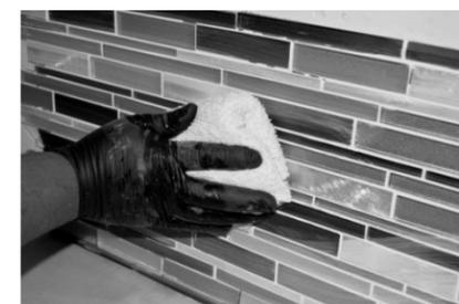
7. Remove spacers once the adhesive has set, prior to grouting. Keep your tools and your workspace clean as you install the tiles. Wipe tiles with a sponge to remove any residual adhesive.
